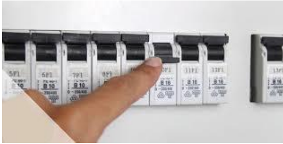
Figure 103: switch on electrical power supply
