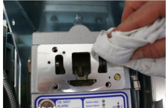
Figure 69: cleaning sealing surface
